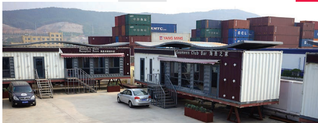
The mobile seafarers' centre in the port of Qingdao has been created with disused containers refurbished into a bar, computer room, reading room, and shops
