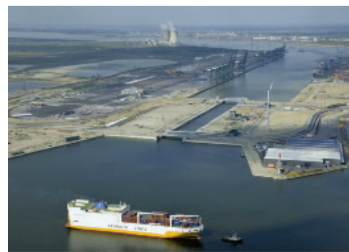
The 71,543gt ro-ro cargo ship Grande Lagos is pictured above becoming the first vessel to use the new Kieldrecht Lock in the Belgian port of Antwerp following its official opening last month. With a length of 500m, a width of 68m and an operational depth of 17.8m, the lock has claimed the title of the largest in the world. Built at a cost of €382m, it is designed to accommodate the largest ships in the world, and to speed up entry into the Waasland harbour. The project took almost five years to complete and is being followed by the Saefinghedok scheme to build a new tidal dock on the left bank of the Scheldt river.
