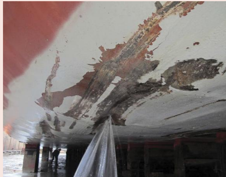
◀ Celtica Hav suffered extensive hull damage, with multiple breaches along its length after grounding in the approaches to the port of Neath Image: MAIB
